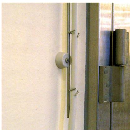
Siltec cable tray for a single cable is especially suitable when conveying a single cable to motors, switches, etc.
