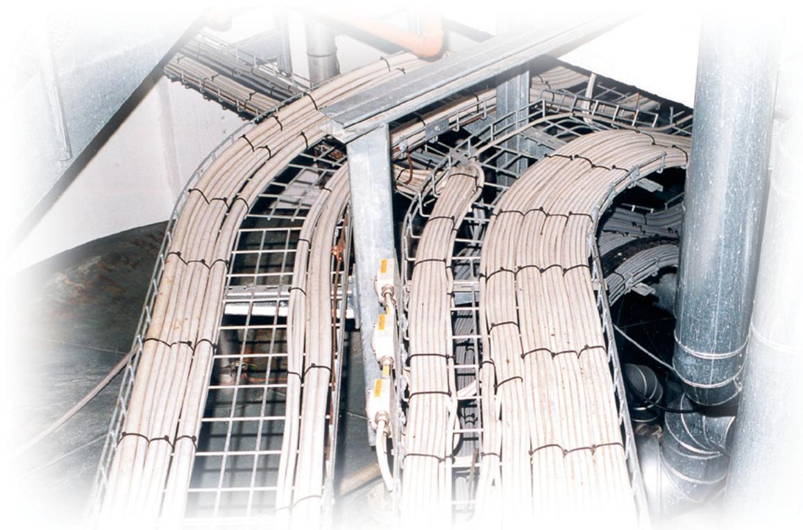
Horizontal and vertical bends can be made from standard cable trays, which simplifies mounting and lowers costs of components.
