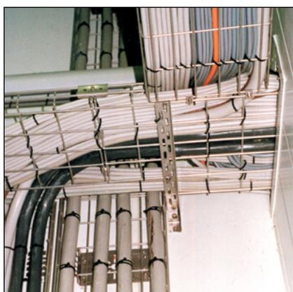
Siltec cable trays are suitable for both thick and thin cables. A grid-spacing of 45 x 86 mm ensures good support and ample room for fixation.
