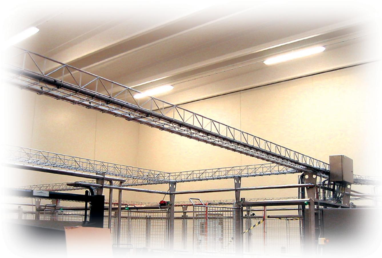
SILTEC heavy-duty cable trays are made with zigzagging longitudinal wires and double side and bottom wires, a combination that ensures a heavy load capacity.
